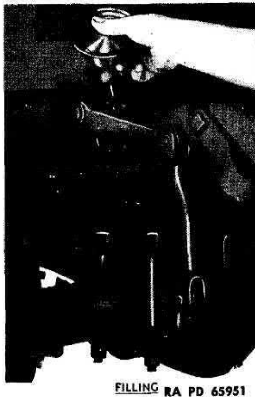
Figure 200—Filling Shock Absorber with Fluid
